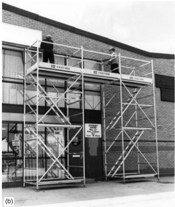
Fig. 10.20 (a) Static tower with stabilising outriggers; and (b) two static towers linked together
