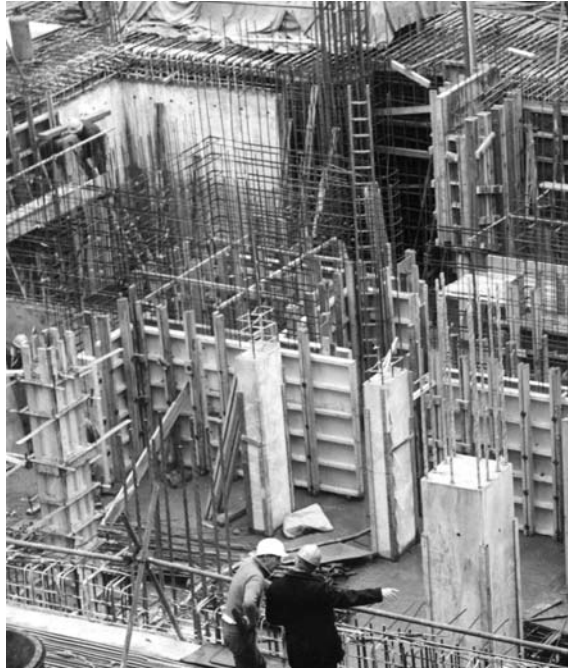
Fig. 3.16 Formwork at different stages of construction
