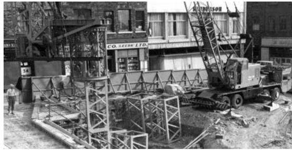
Fig. 2.13 Hoarding viewed from inside a city-centre building site
