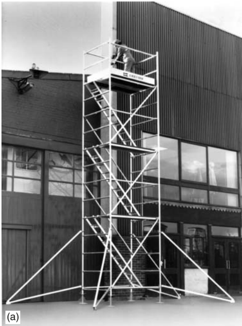
Fig. 10.20 (a) Static tower with stabilising outriggers; and (b) two static towers linked together
