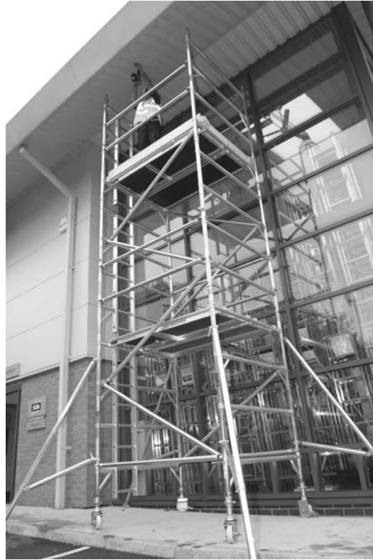
Fig. 10.19 SGB mobile tower
