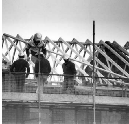
Fig. 8.28 Trussed-rafter roof being erected
