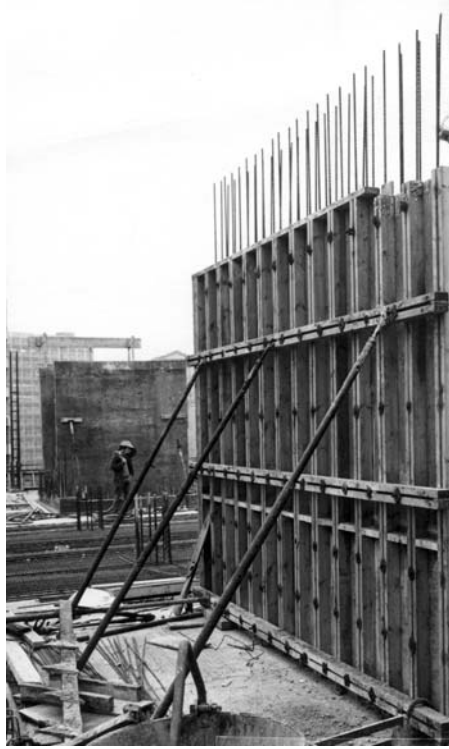
Fig. 3.13 Erection of wall form
