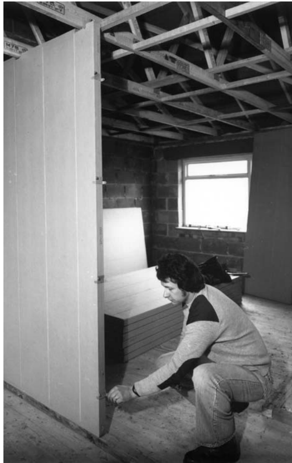
Fig. 9.14 Installing a 'Karpfos' partitioning system
